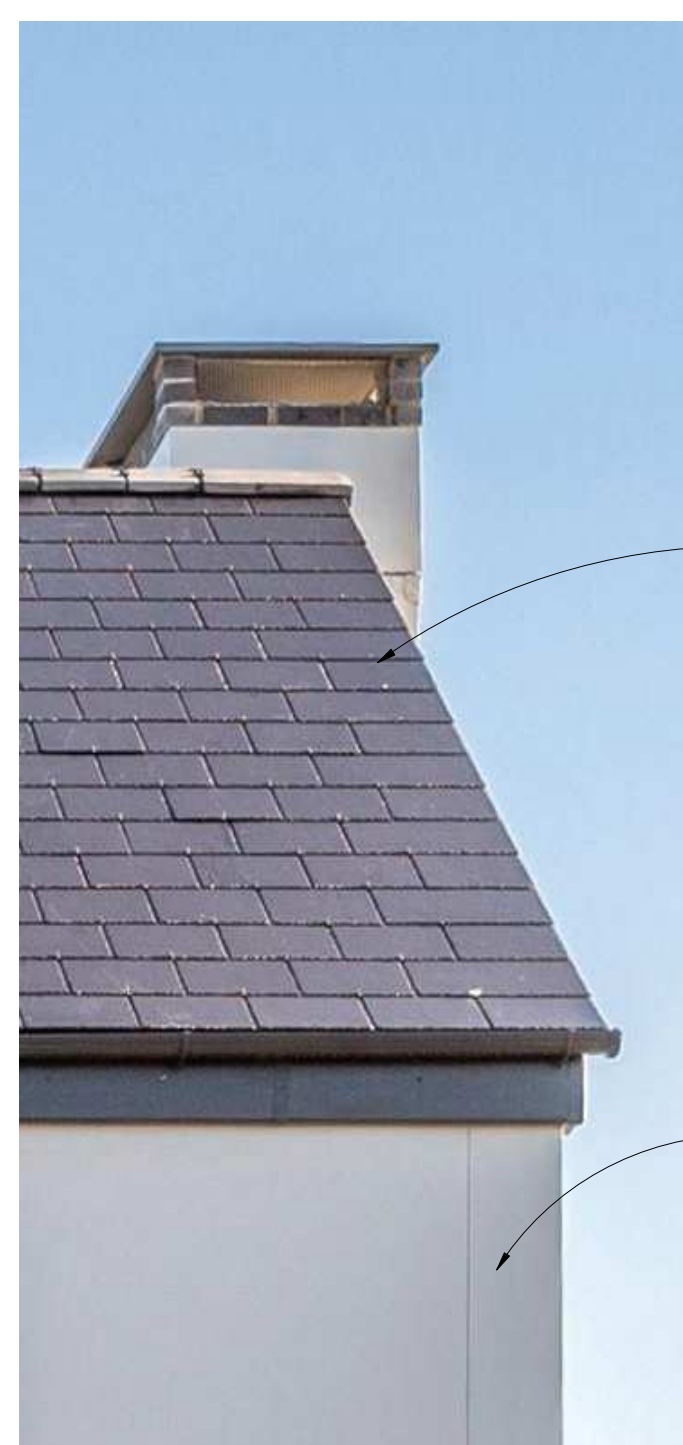
Natural Slate Roofing
