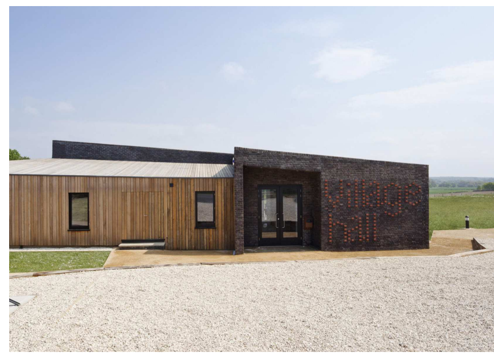
Barcombe Village Hall - The utilisation of differing materials to the roof pitches depicts the divide in functions.
