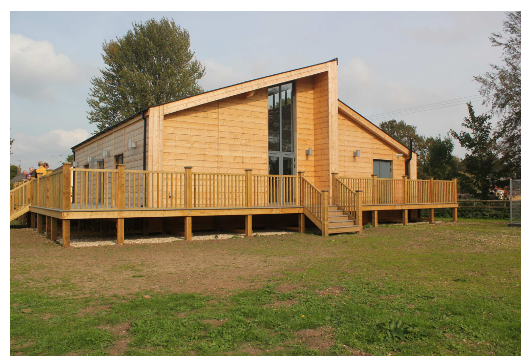
Stourpaine Village Hall - The use of two projecting offline and timber cladding, making this an economical
